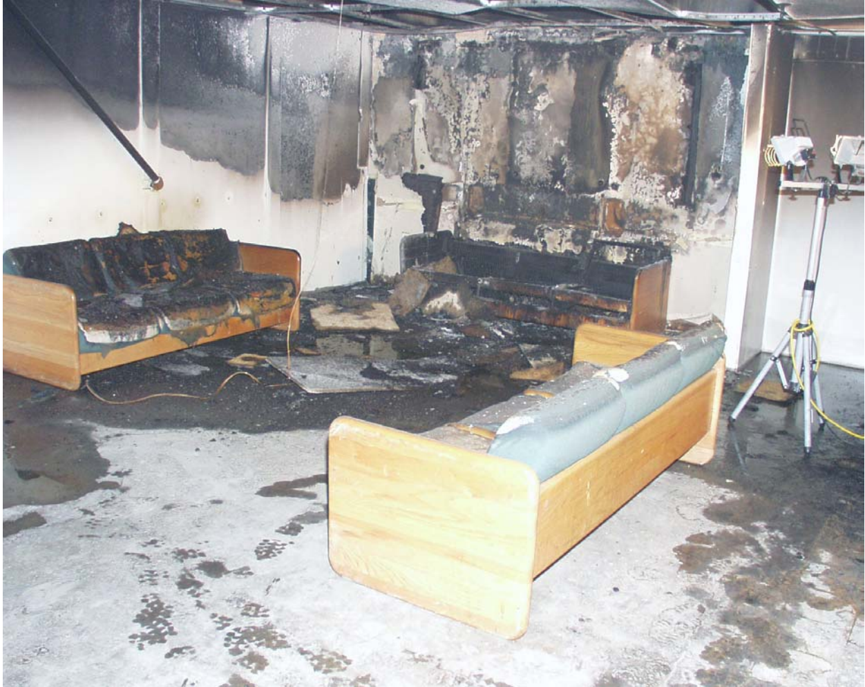
Figure 13. Photograph showing the day room after experiment 2.
