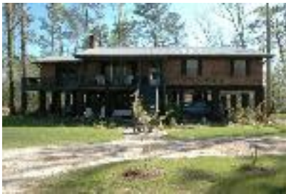
The Palmers' elevated brick house.
