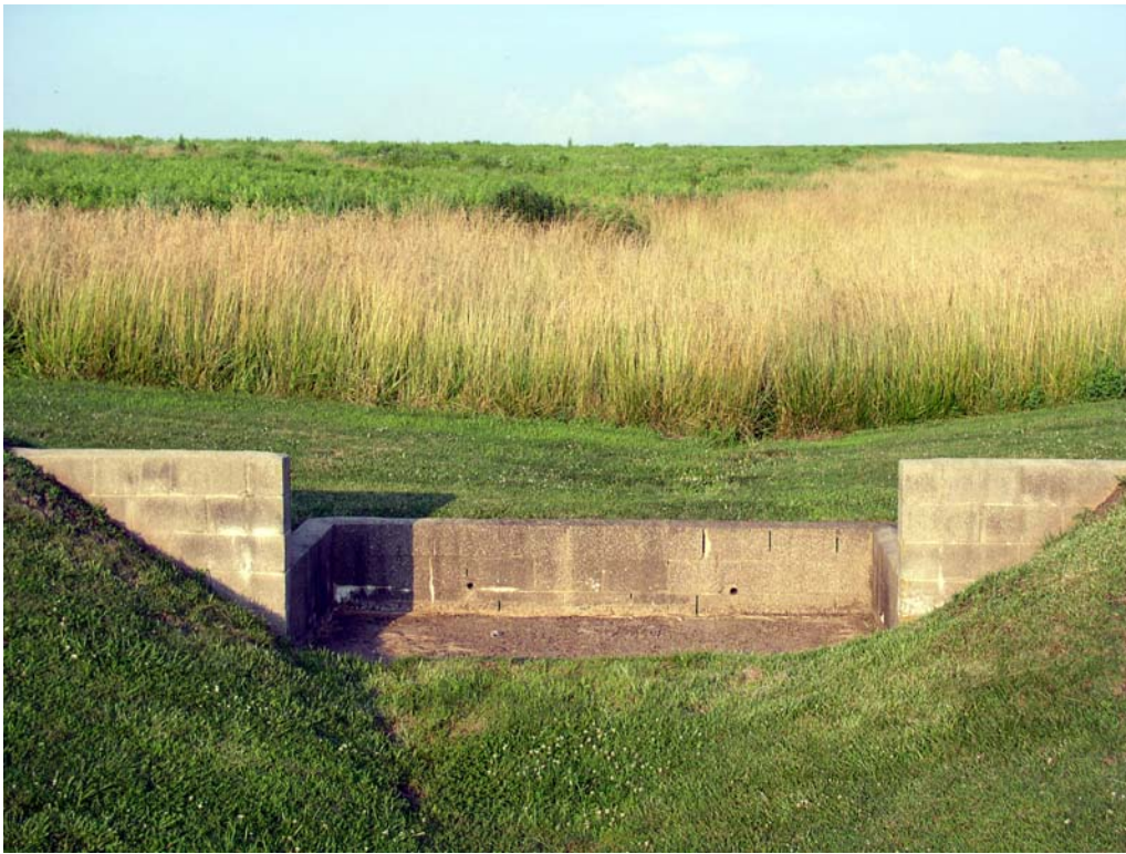
Figure 16.—A grade-stabilization structure prevents gullying at this grassed waterway outlet in an area of Atlas soils.
