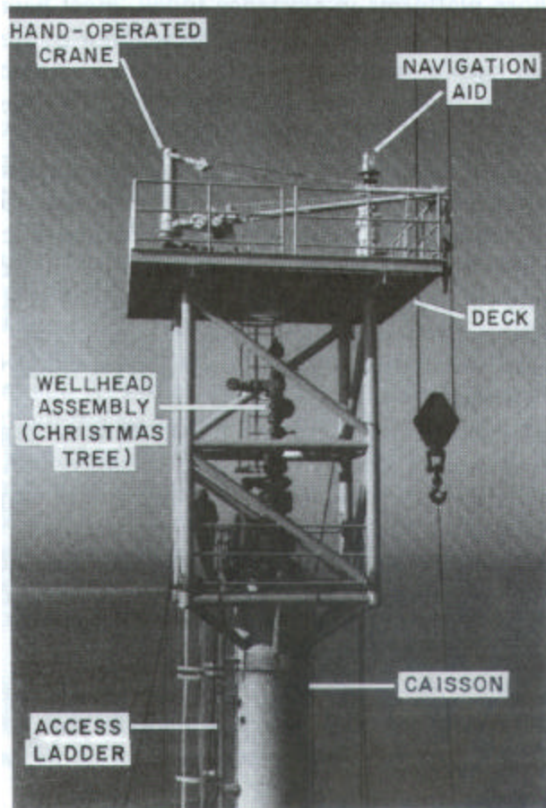
Figure 1-2. Typical caisson well-guard platform. [Drawe and Riefel, Ed. McClelland and Riefel, Copyright © 1986 by Van Nostrand Reinhold Co., Inc.]
