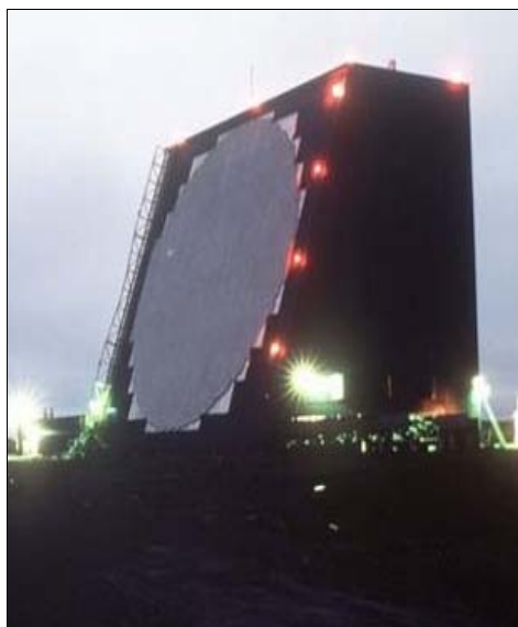
Figure 1. AN/FPS-108 Cobra Dane L-band phased array radar.
