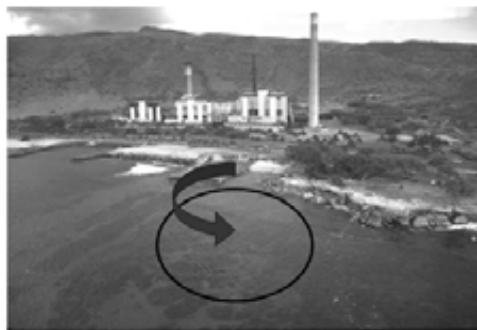
Kahe Point Electric Generating Station, Oahu, Hawaii
