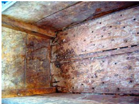
Box with drilled holes in floorboards
