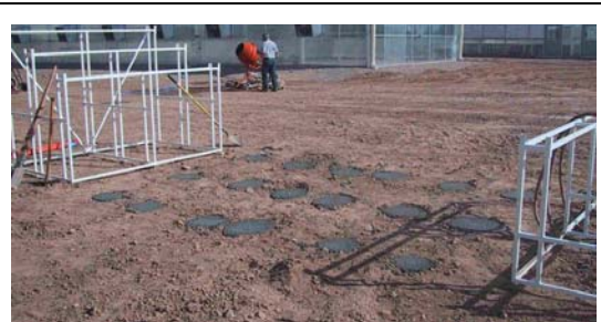
Figure 3. Nine small concrete pads to support the steel frame.
