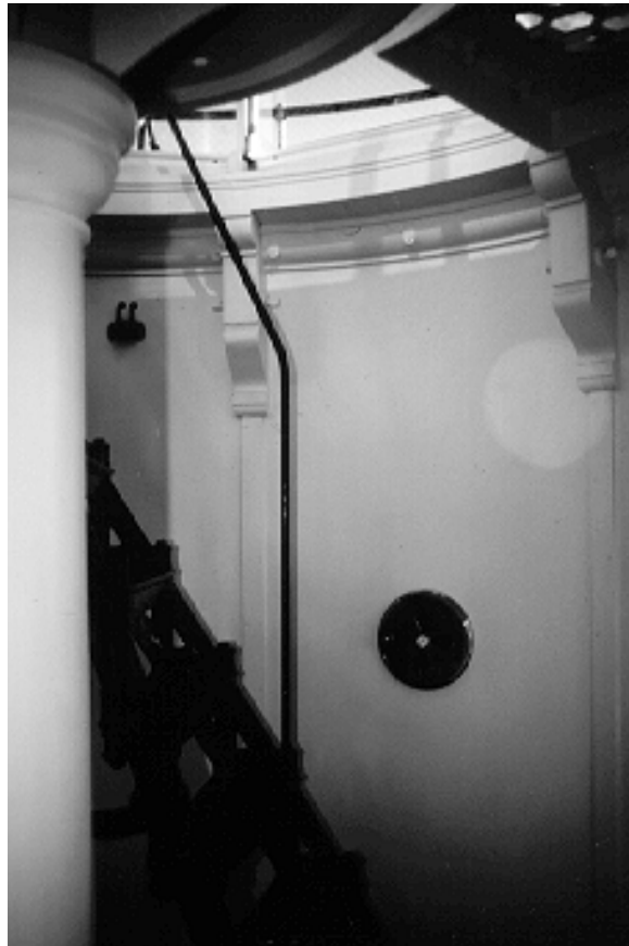
Figure 38. Service room bracket after chemical cleaning.
