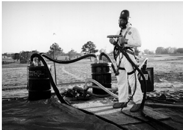
Figure 29. Worker dressed in full personal protective gear. The full-face-shield self-contained respirator provides both respiratory and eye protection. The worker is wearing protective coveralls, gloves, and boot covers to prevent lead dust contact. The harness is part of a full protection system. He is holding a pneumatic needle gun that is hooked to a two-stage HEPA (High Efficiency Particulate Air) filtered vacuum system.
