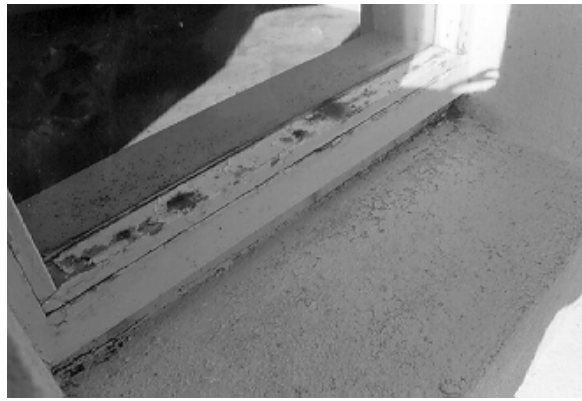
Figure 26. This steel casement window frame was not sealed properly and as a result has begun rusting from the inside out.
