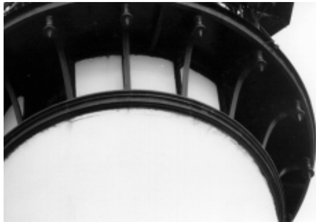
Figure 41 (left). This masonry lighthouse has been detailed with a two-tier cast-iron water table (the iron portions are painted black). Rust-bleed is occurring along lower edge of the upper tier.
