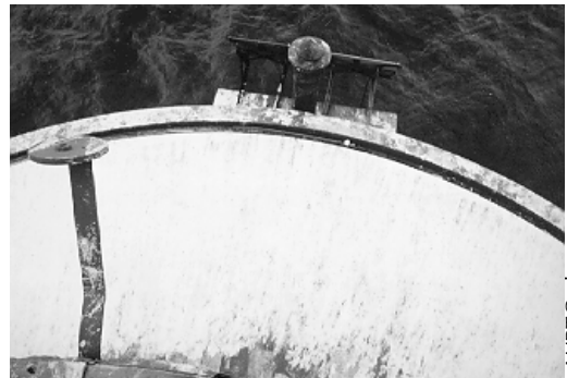
Figure 22. Interior of a sheet-iron parapet wall that is rusting from the inside to out along the lantern room door. This is the result of water entering the interior cavity of the parapet wall.
