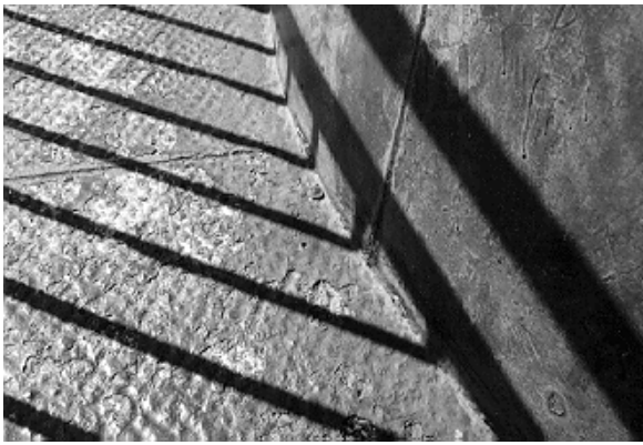
Figure 25. The seams between the deck and wall plates of this lighthouse were not properly sealed; as a result the areas collected water and began to rust.
