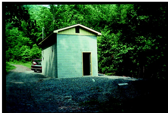
Figure 9-4. New cinder block building.
