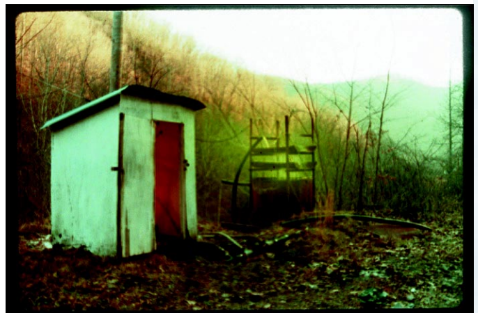
Figure 9-2. Old treatment system.
