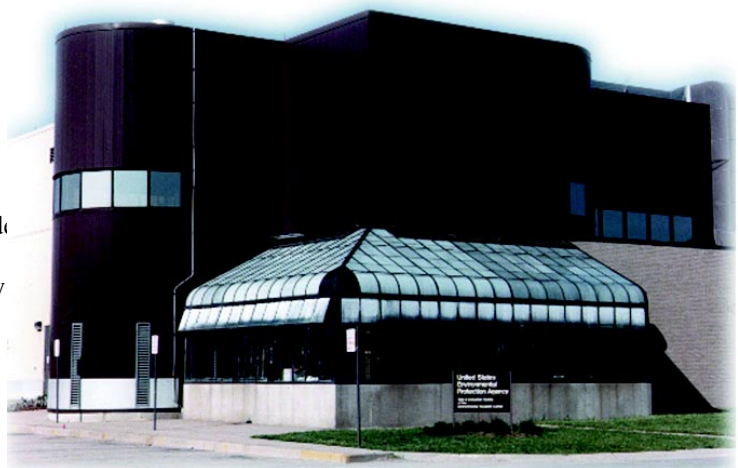
Figure 1-1. EPA Test & Evaluation Facility, Cincinnati, OH.
