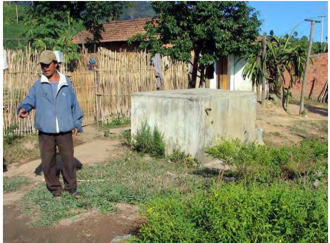
No Longer Functioning UNICEF Water Tank
