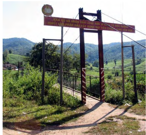
Foot Bridge over Stream
