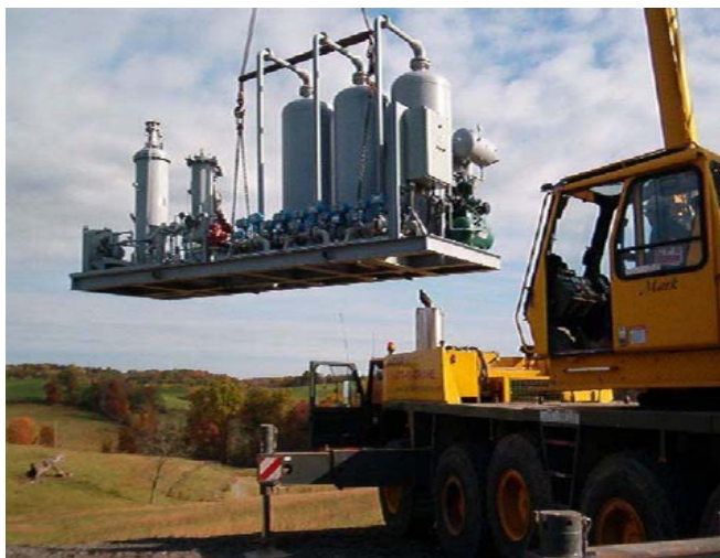
Figure 5. The footprint of this small, nitrogen removal unit is 8 by 25 feet, with vessels, vacuum pump, instrument air system, valves, and instrumentation atop. (Compression unit and other peripheral items are not shown.) This skid weights about 25,000 pounds and is shipped on a double-drop truck. A crane is needed for installation.
