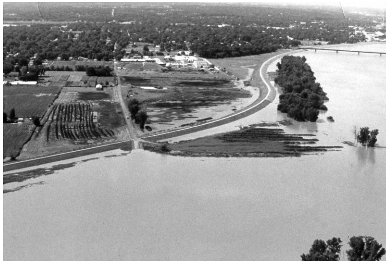
FIGURE 9-1: Levee on Kansas River
