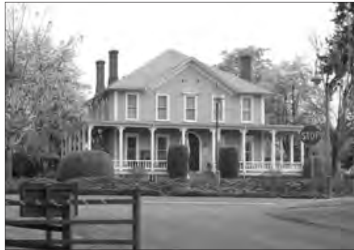
Officers' Row residences and Barracks buildings dating from this historic period are predominantly the oldest structures in the Reserve.
