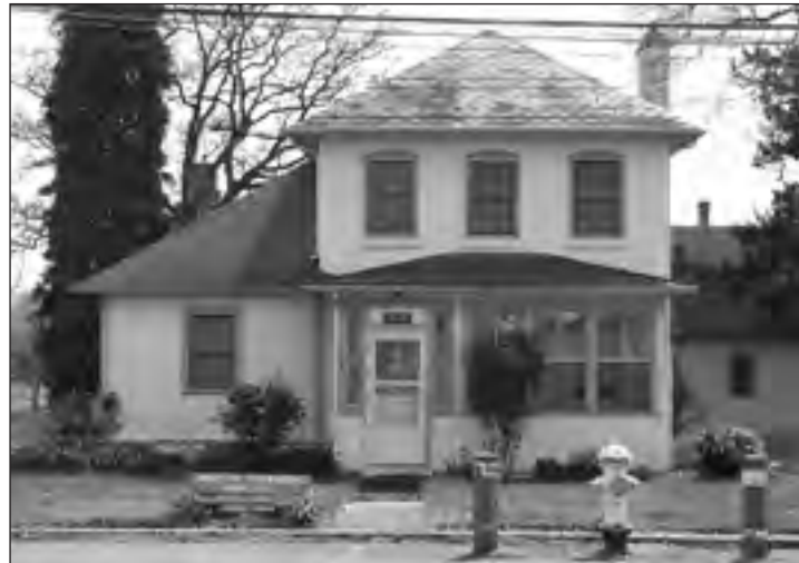
Hospital Steward's Quarters was constructed in 1907.
