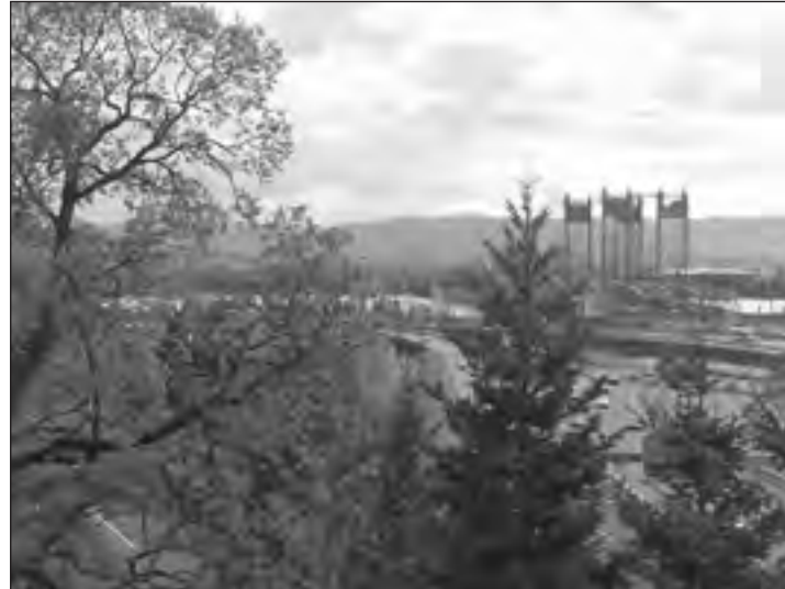
Construction of Interstate 5 and its bridge over the Columbia River severed the direct connection between the West Barracks and the City of Vancouver.
