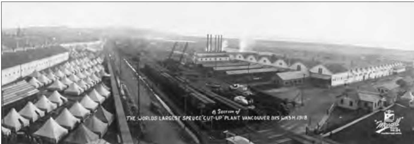
Spruce Production Plant, one of the world’s largest spruce cut-up plants, employed 30,000 work soldiers to produce up to one million board feet of lumber a day.
