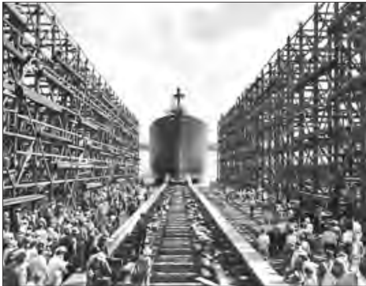
One hundred forty-one military ships were constructed rapidly and launched in 44 months due to Kaiser's innovative assembly-line production methods. Eleanor Roosevelt christened the shipyard's first aircraft carrier Alazon Bay in April 1943.
