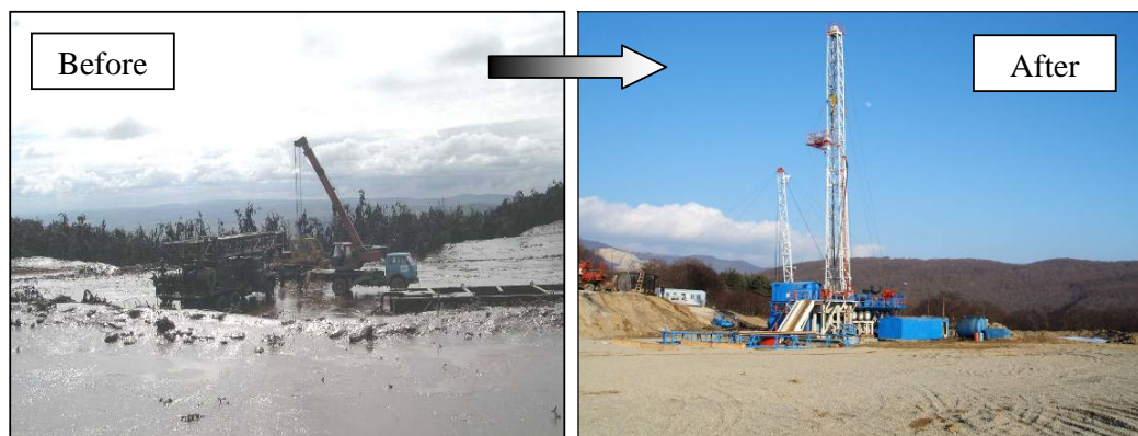
Figure 3. Showing the wellhead site immediately after the spill and four months after.
