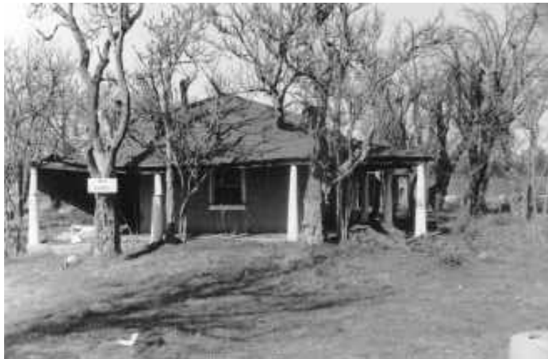
South-facing elevation of original Jose Maria Gil Adobe (c. 1865) constructed on El Camino Real, overlooking San Antonio River. Ranch residence until 1940; served through 1950s as Bachelor Officers' Quarters. Pending restoration, structure is "moth-balled." Courtesy U.S. Army, FHL Archives, 1979.
