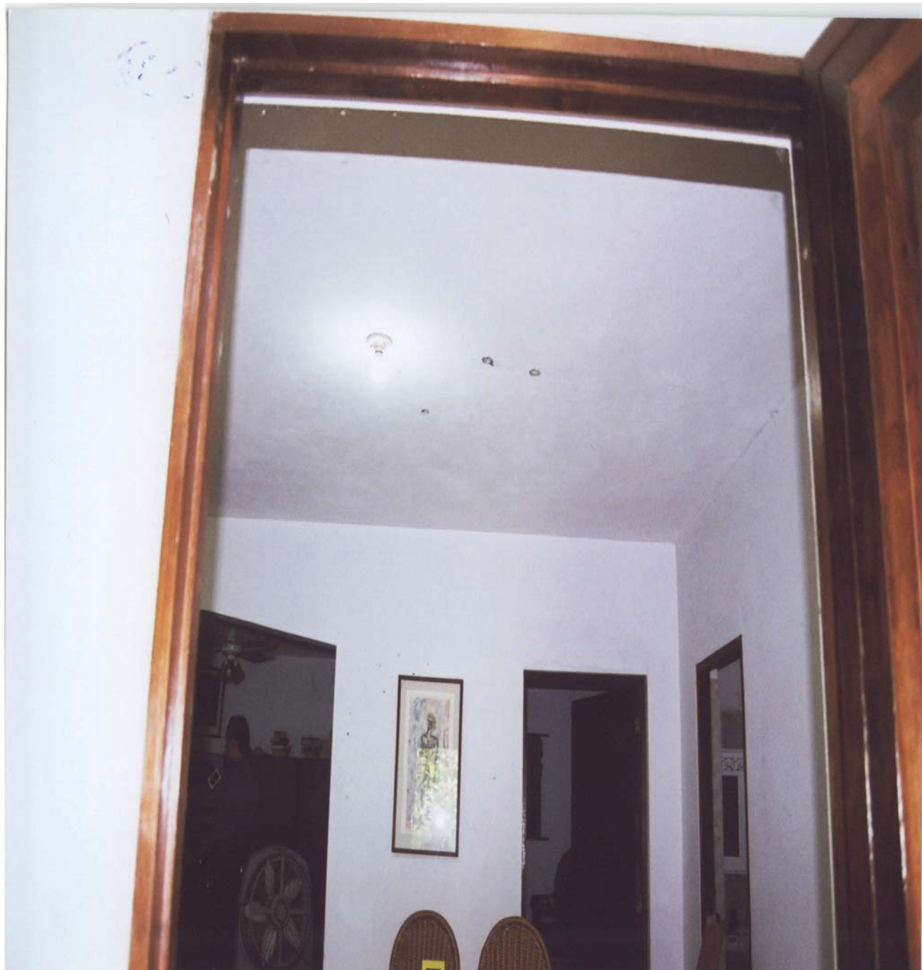
FIGURE 13 Ceiling Impacts from Shots Through Front Door
