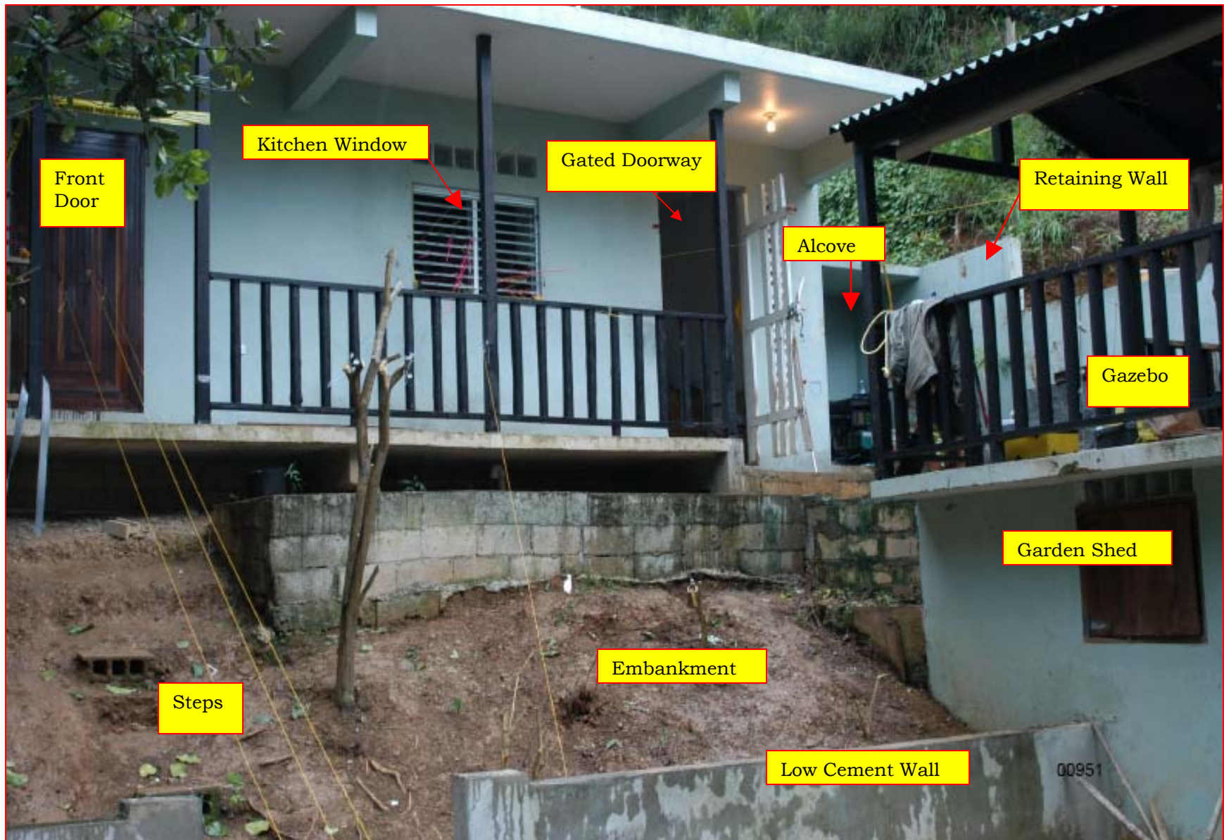
FIGURE 6 Selected Features on Front (White) Side of Residence (Foliage Removed)
