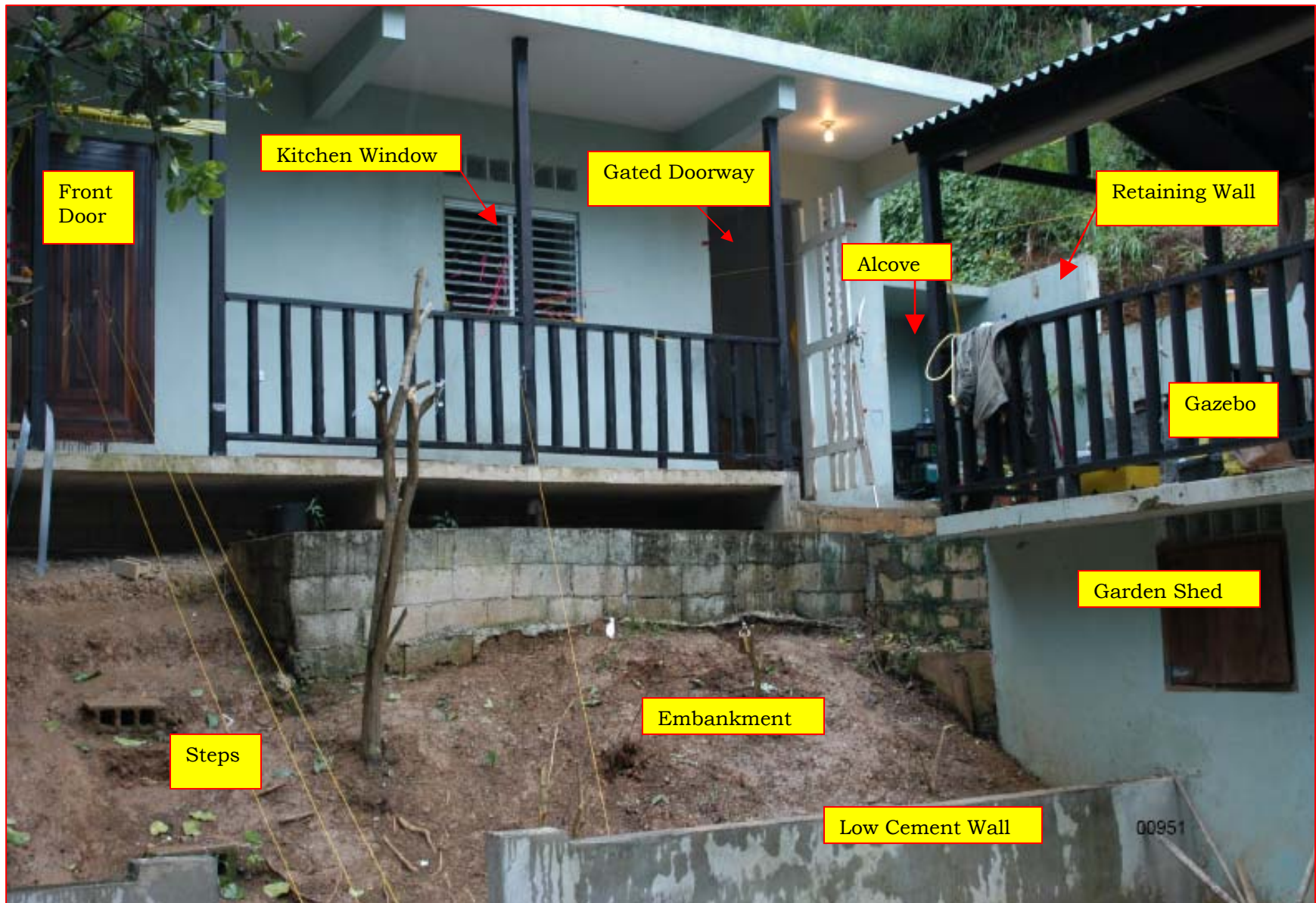
FIGURE B Selected Features on Front (White) Side of Residence (Foliage Removed)
