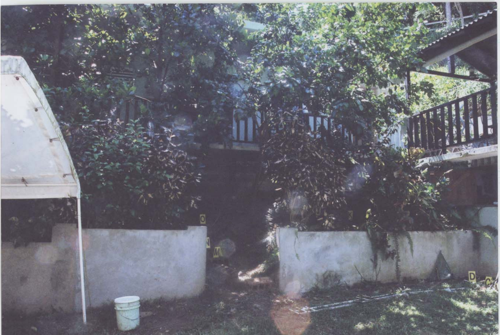
FIGURE 8 View of the Front of the Residence (Before Foliage Removed)
