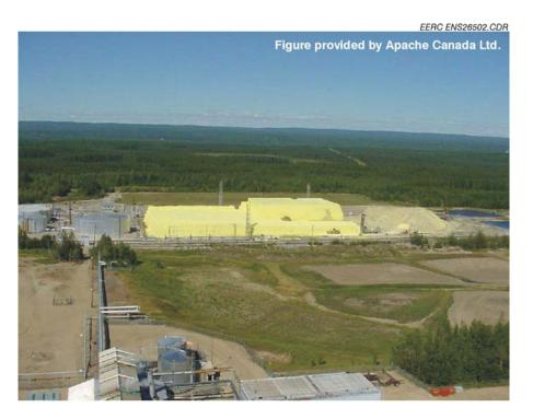
Figure 3. Elemental sulfur accumulating as a result of acid gas processing.
