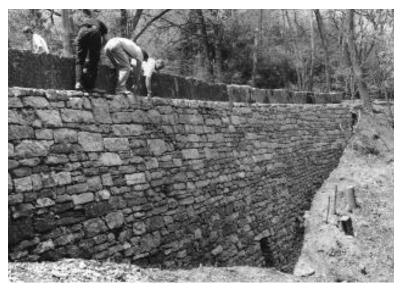
The park wall was completely dismantled and authentically rebuilt at a savings of \$100,000 over the bid for a concrete replacement.
