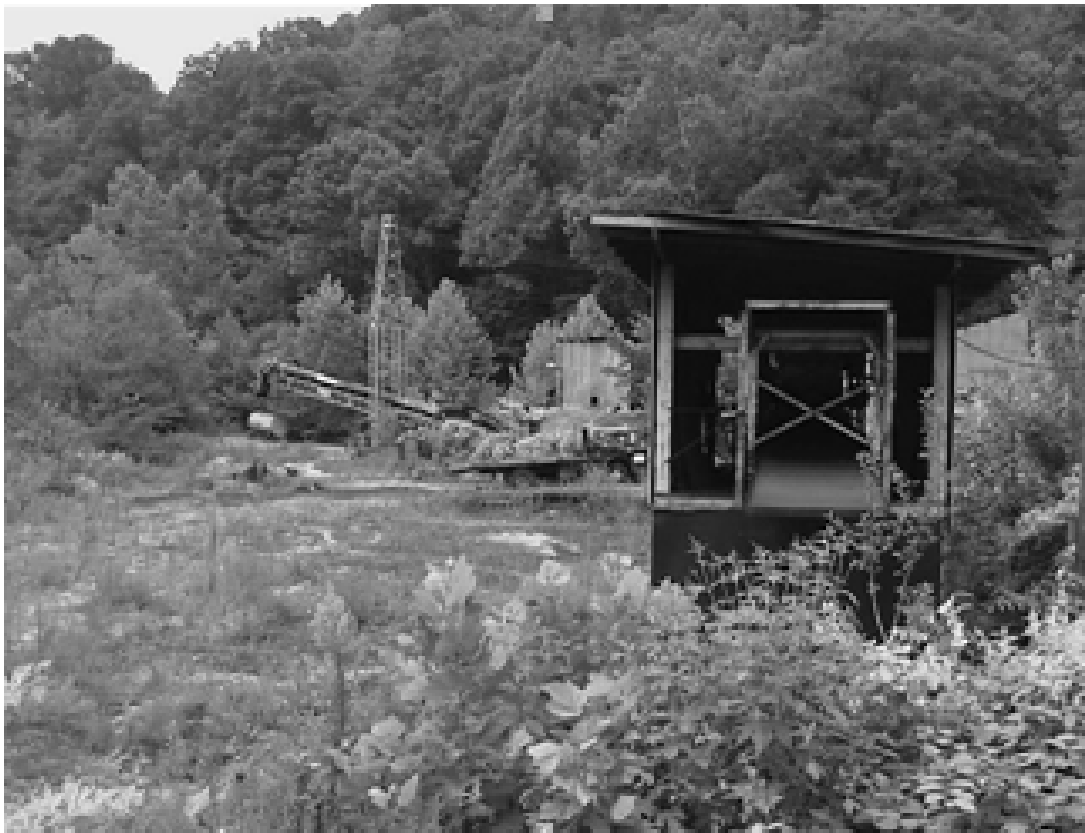
Stone Creek Tipple Site
