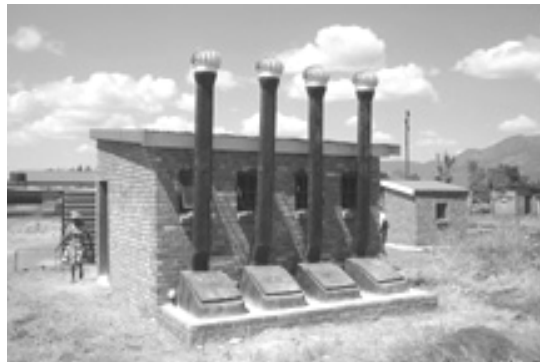
An "enviroloo" (dry composting toilets) mandated by the Department of Public Works in the Northern Province of the Republic of South Africa (2002)
