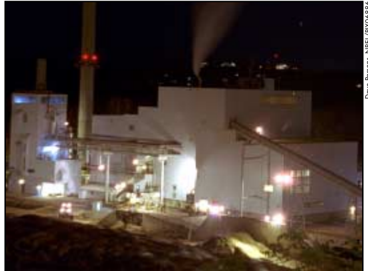
The McNeil Generating Station at night
