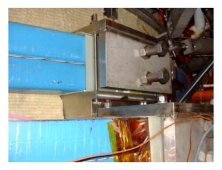
There are six pads per coil, and four 1/2"-13 threaded rods per clamp. An important feature to note is that, while the stud end away from the midplane is attached via a nut, the opposite end is threaded into the base metal where it is 3/4" thick. Due to limited space, nuts and washers are not feasible. The pads are welded to the VV (not visible in the photo above, hidden behind the thermal insulation).
