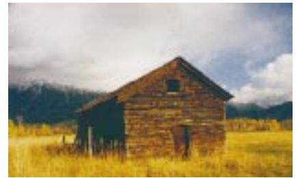
OLD BUILDINGS CAN BE USED FOR NURSERY ROOSTS. Mitchell Firman photo
