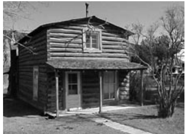
The historic mail carrier's house will receive much-needed stabilization.
