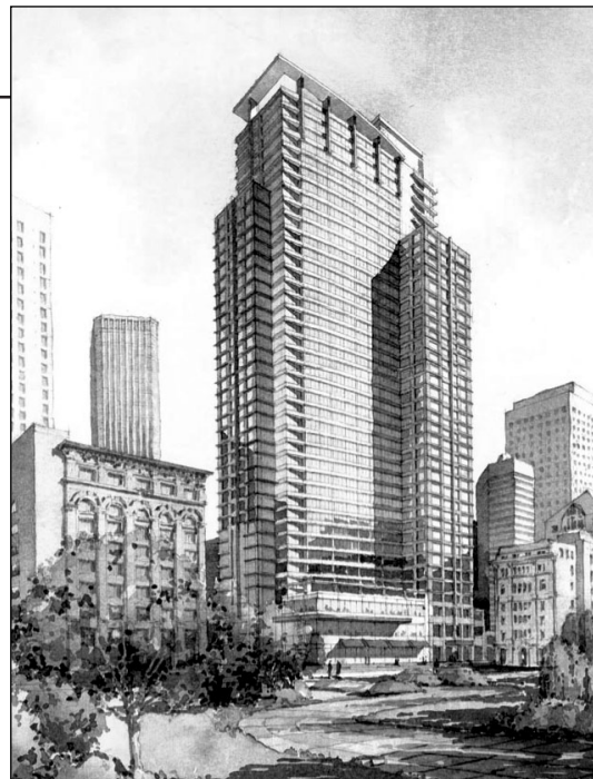
Thirty-nine-story precast concrete building in San Francisco.
