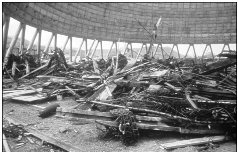
Collapse of a portion of a reinforced concrete hyperbolic cooling tower.
