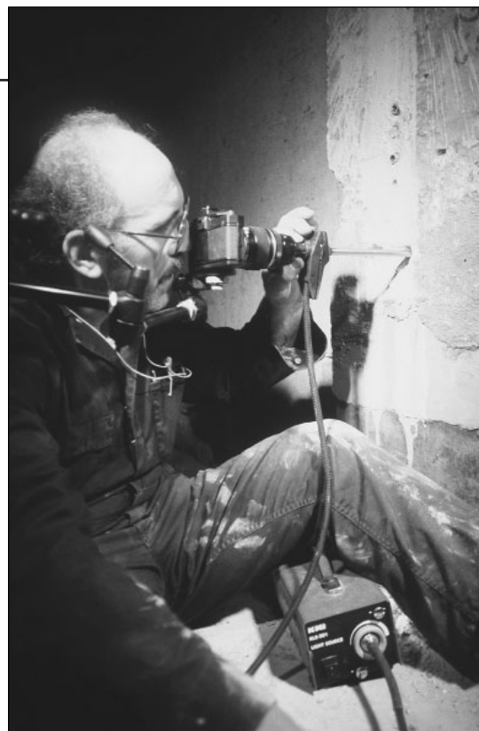
CBT investigator Nicholas Carino, research structural engineer, uses a borescope to examine the condition of the joint between segments of precast columns in the U.S. Embassy Office Building in Moscow. The investigation revealed many cases where large voids were present in the joints between precast structural members.
