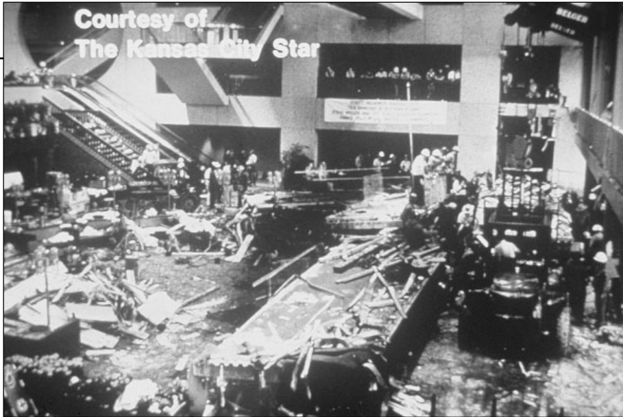
Collapsed walkways in the Hyatt Regency Hotel atrium.
