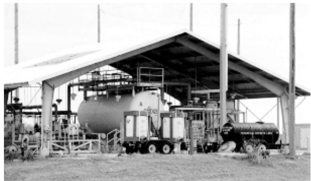
The Nitrogen Tetroxide Scrubber has been installed in the Oxidizer Farm at Launch Pad 39A.
