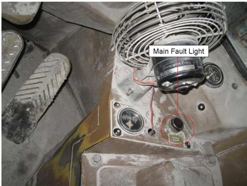
PHOTO No. 2: Main Fault Light in the Forward Right Area of the Operator's Compartment
