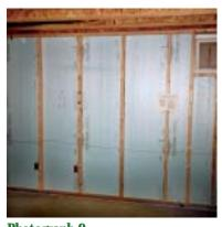
**Photograph 9**Unfaced extruded polystyrene against basement wall
