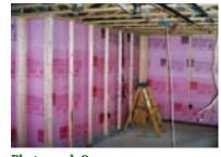
**Photograph 8**Unfaced extruded polystyrene against basement wall
