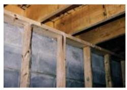
**Photograph 1**Interior stud framing located at basement perimeter
