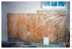
**Photograph 5**Frame wall with interior vapor barrier resulting in mold, decay and odors
