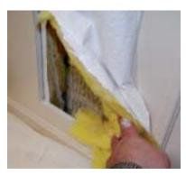
**Photograph 7**Mold with blanket insulation
