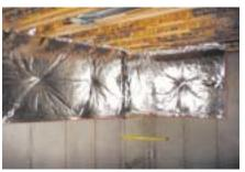
**Photograph 4**Blanket insulation with impermeable aluminum foil interior surface
