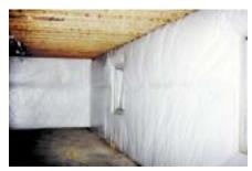
**Photograph 3**Blanket insulation with impermeable vinyl interior surface
