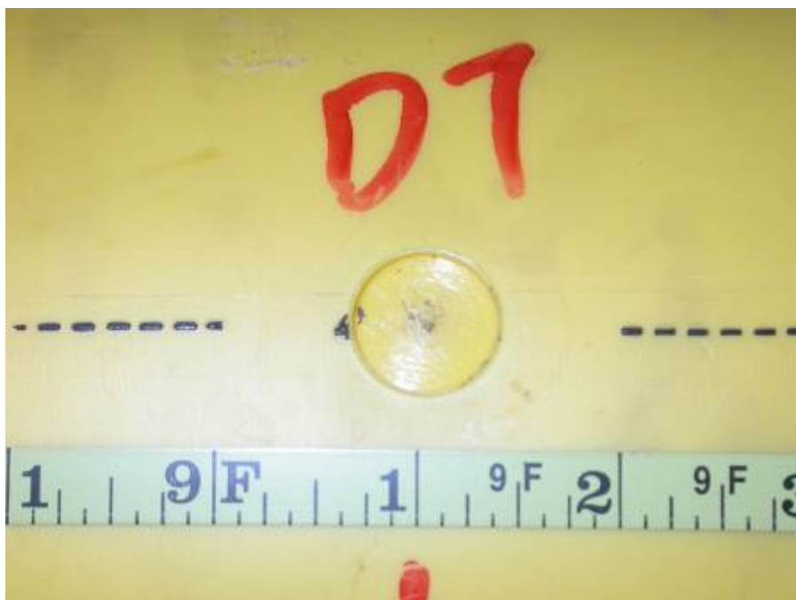
Figure 5-9. Defect D13 (D7)
