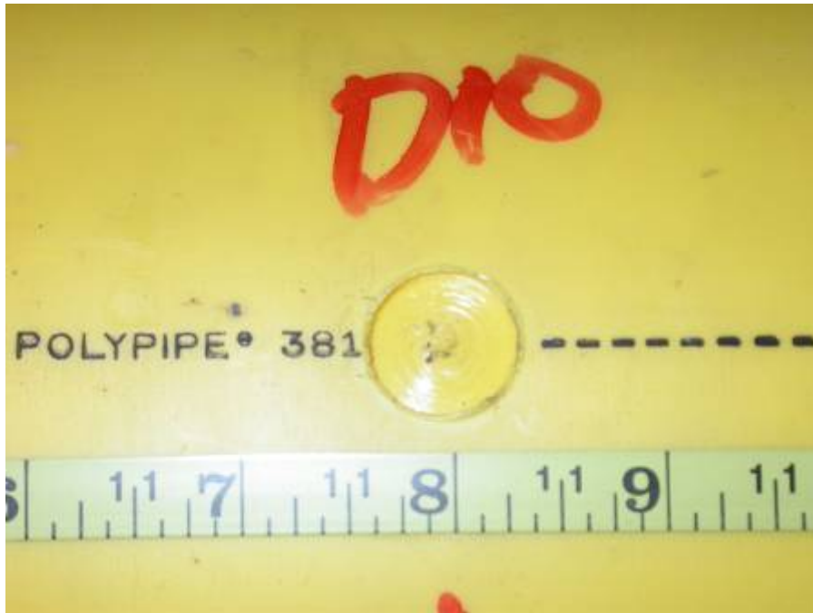
Figure 5-12. Defect D18 (D10)
