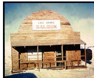
Photo by Bob Nyden / Special to The Antarctic Sun Seabees built the Last Chance Saloon from packing crates.
