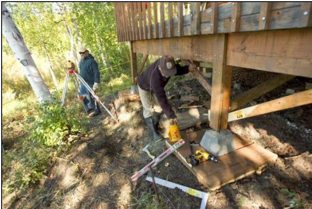
Maintenance Worker Holton (rear) and Wildlife Biologist Akaran (Yukon Flats NWR) overhauled the Kanuti Cabin's foundational structure. The cabin is now level for the first time in many years. (S. Hillebrand photo)
