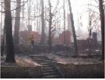
The remains of the Mt. Lemmon Domestic Water Improvement District Manager's home following the Aspen Fire
