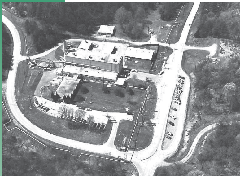
Aerial view of the Molten Salt Reactor Experiment site in Melton Valley.
