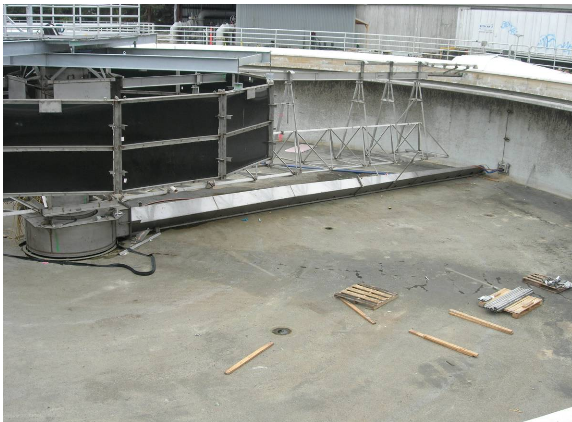
Secondary clarifiers undergoing upgrade construction at LOTT's Budd Inlet Treatment Plant (2006)
