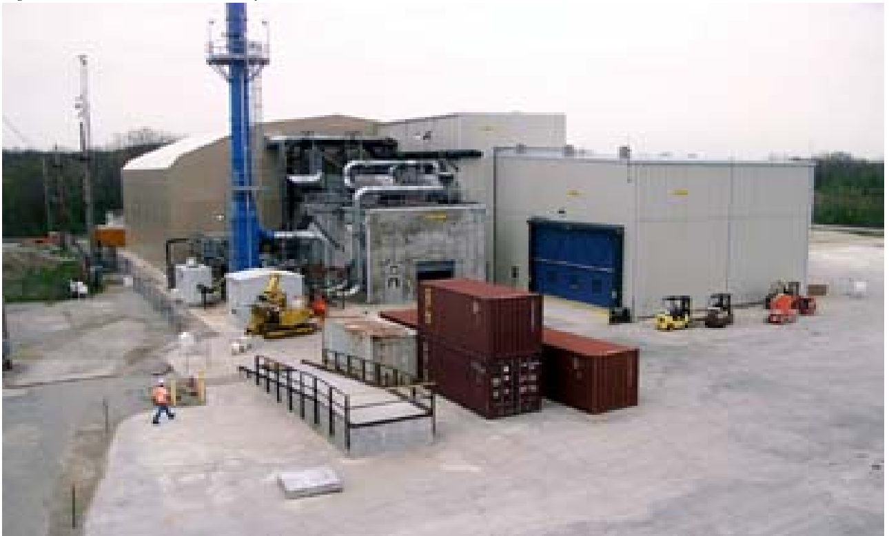
Figure G-3 Silo 3 Remediation Facility
