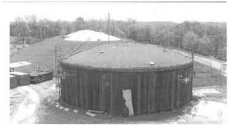
Silo 3 contains 5,088 cubic yards of uranium processing residues
