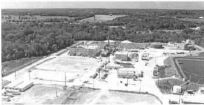
The Silos 1&2 and Silo 3 project area
