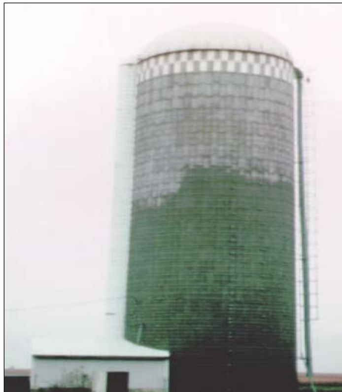
Color differences indicate area dried due to heat of fire
