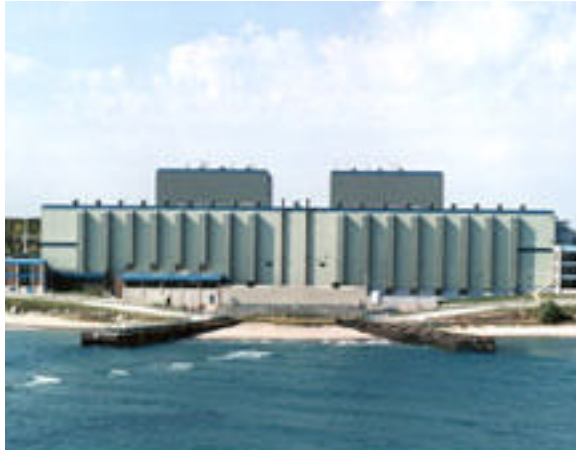
Point Beach Nuclear power Plant, Two Creeks, Wisconsin
