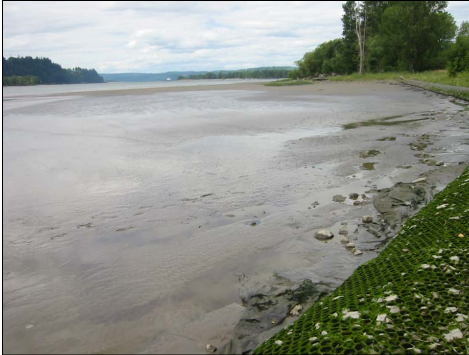
Figure A-3. Barlow Point, upstream end of site. The upper part of the beach is protected by a gabion structure known as "Reno mat."
