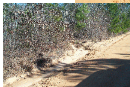
Turn-outs into filtering areas.
