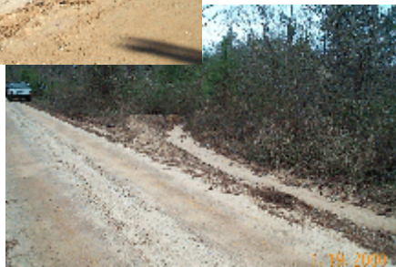
Turn-outs into filtering areas.
