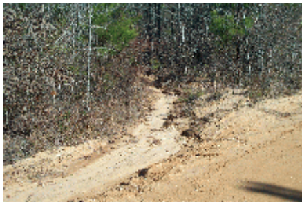
Turn-out to a drop inlet.
