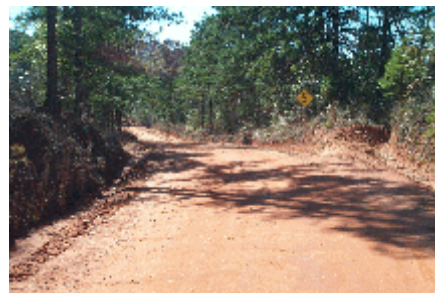
Turn-out at gradient changes.
