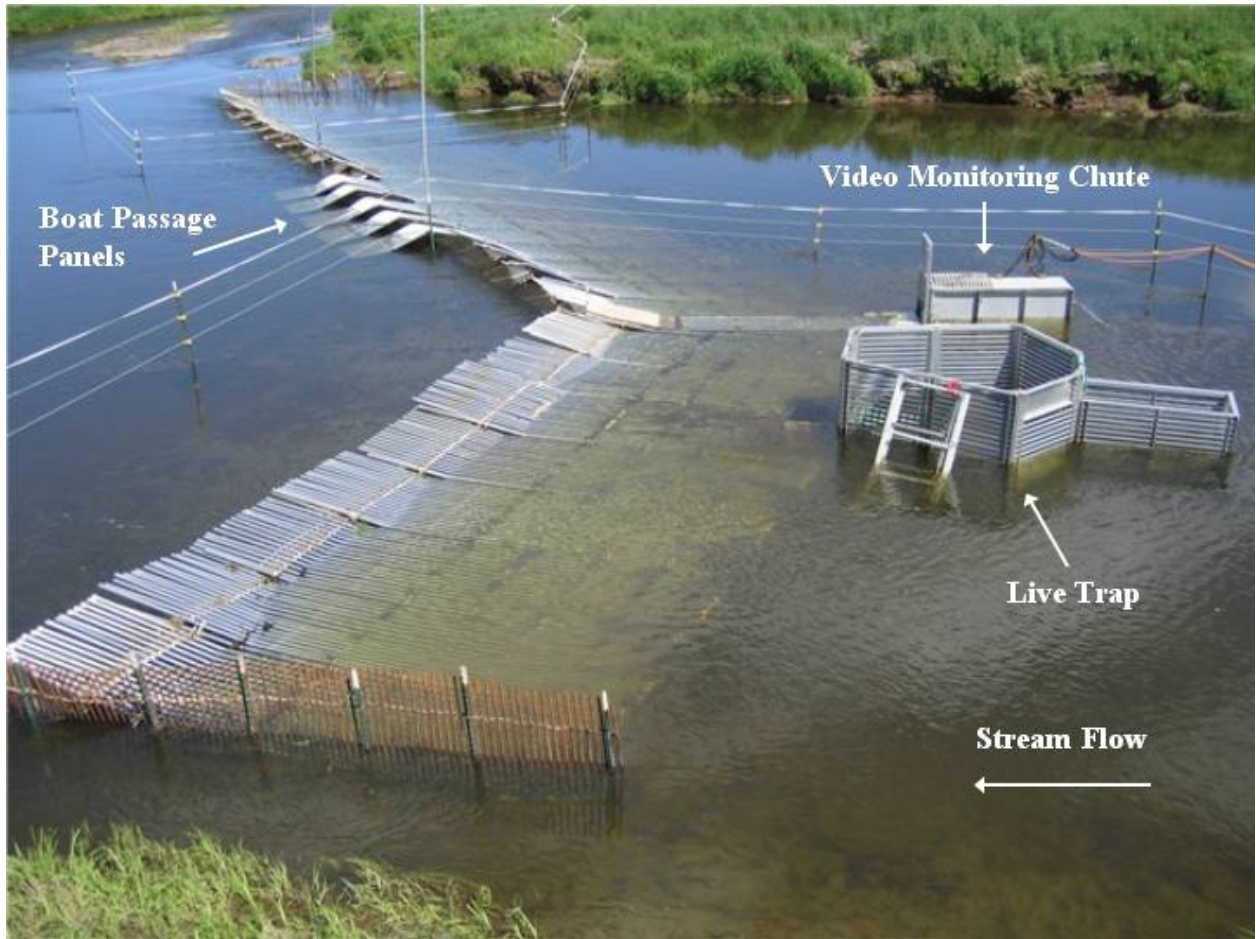
Figure 2. Overview of the V-shaped resistance board weir used at Big Creek from 2002 to 2004.
