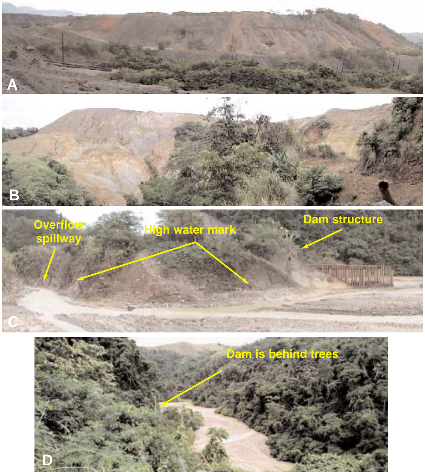
Figure 6. A. Mine dump that was used as an acid leach dump for copper extraction. B. Mine dump north of the San Antonio pit above the Maguila-guila siltation dam. The yellow-to-orange colors on the dump indicate the presence of secondary salts, which show that sulfide-rich rocks (gray) are generating acid drainage. C. The Maguila-guila siltation dam, downstream from the dump shown in B, no longer fulfills its purpose to trap sediment eroded from the mine site. Sediment has completely filled the ~25 (?) m high impoundment and water is now flowing out the overflow spillway. Note the high-water mark on the dam, indicating that the overflow spillway is not big enough to prevent debris buildup and backup of waters during high stream flows. D. Looking north at sediment trapped behind the Maguila-guila dam.
