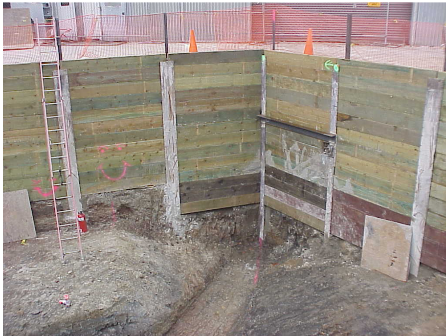
Southeast corner of the excavation – September 28, 2006.
