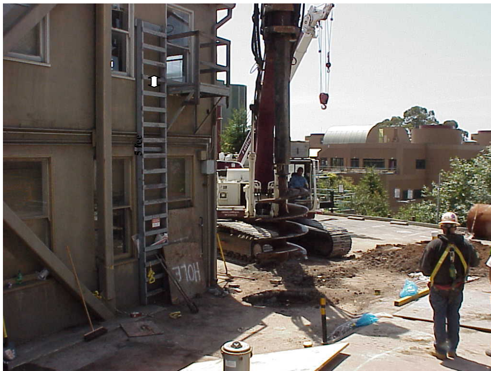
Initial boring using 48" augers at northwest corner of Building 7 – April 15, 2006
