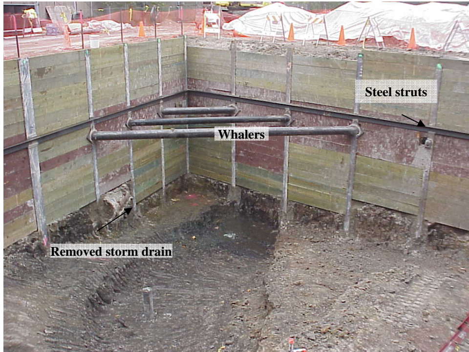
Northwest corner of excavation – September 28, 2006.
