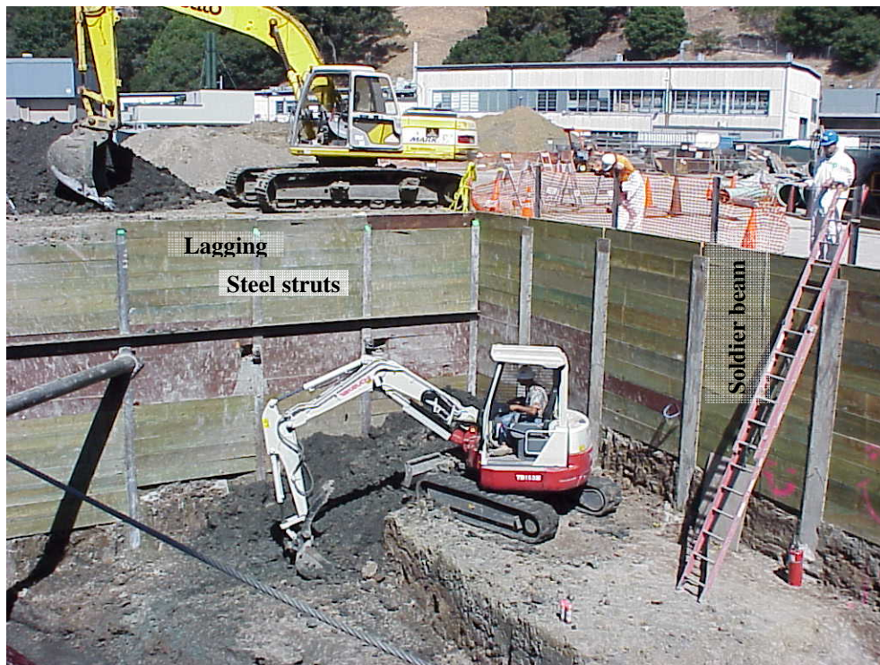
Northeast corner of excavation - September 21, 2006.
