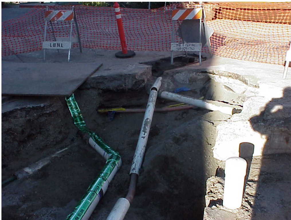
Former Building 7 Sump Excavation
