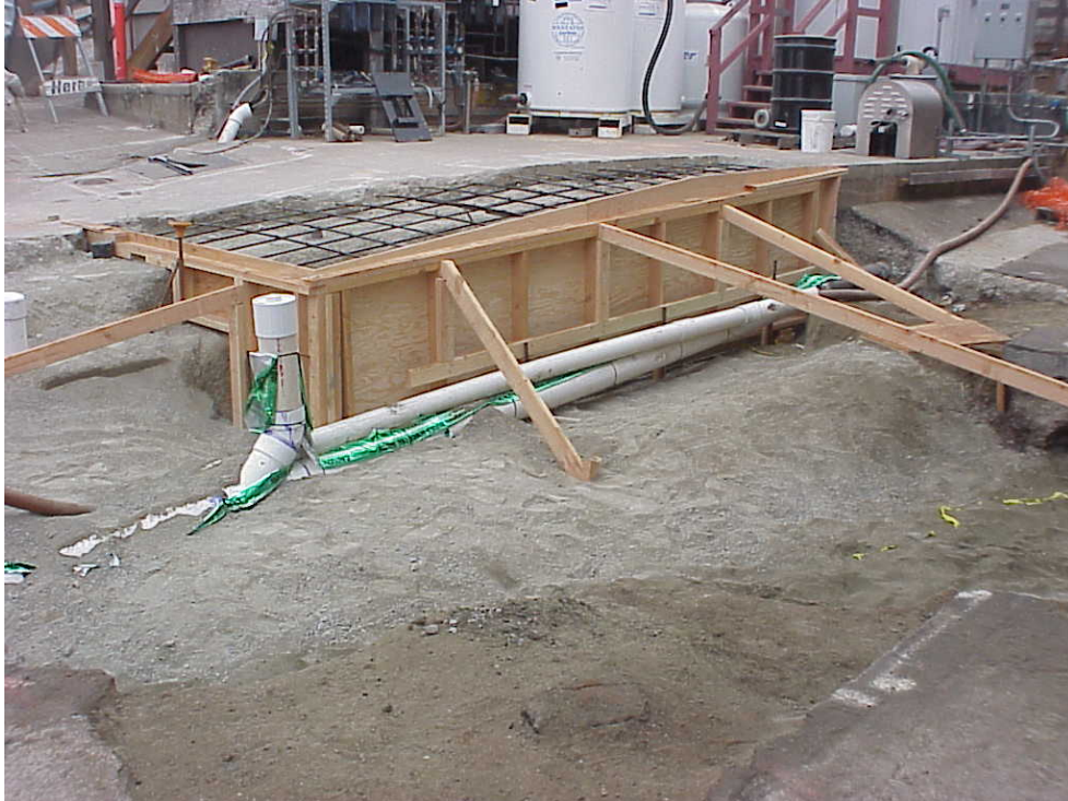
Post-excavation utility and surface restoration- September 28, 2006.
