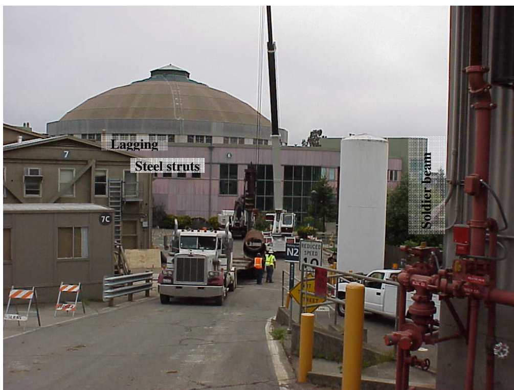
Preparing temporary casings - September 21, 2006.
