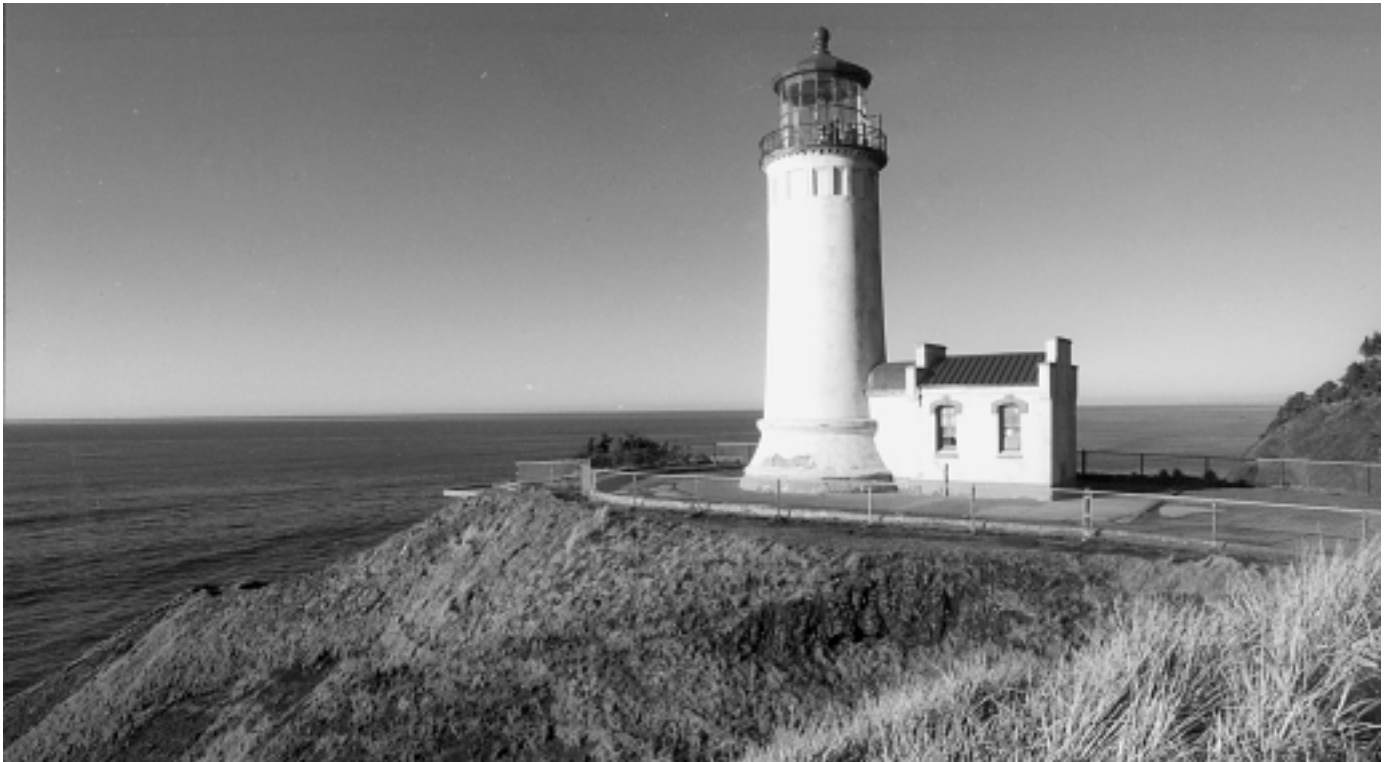
North Head Lighthouse (1898) near Ilwaco, Wash.
