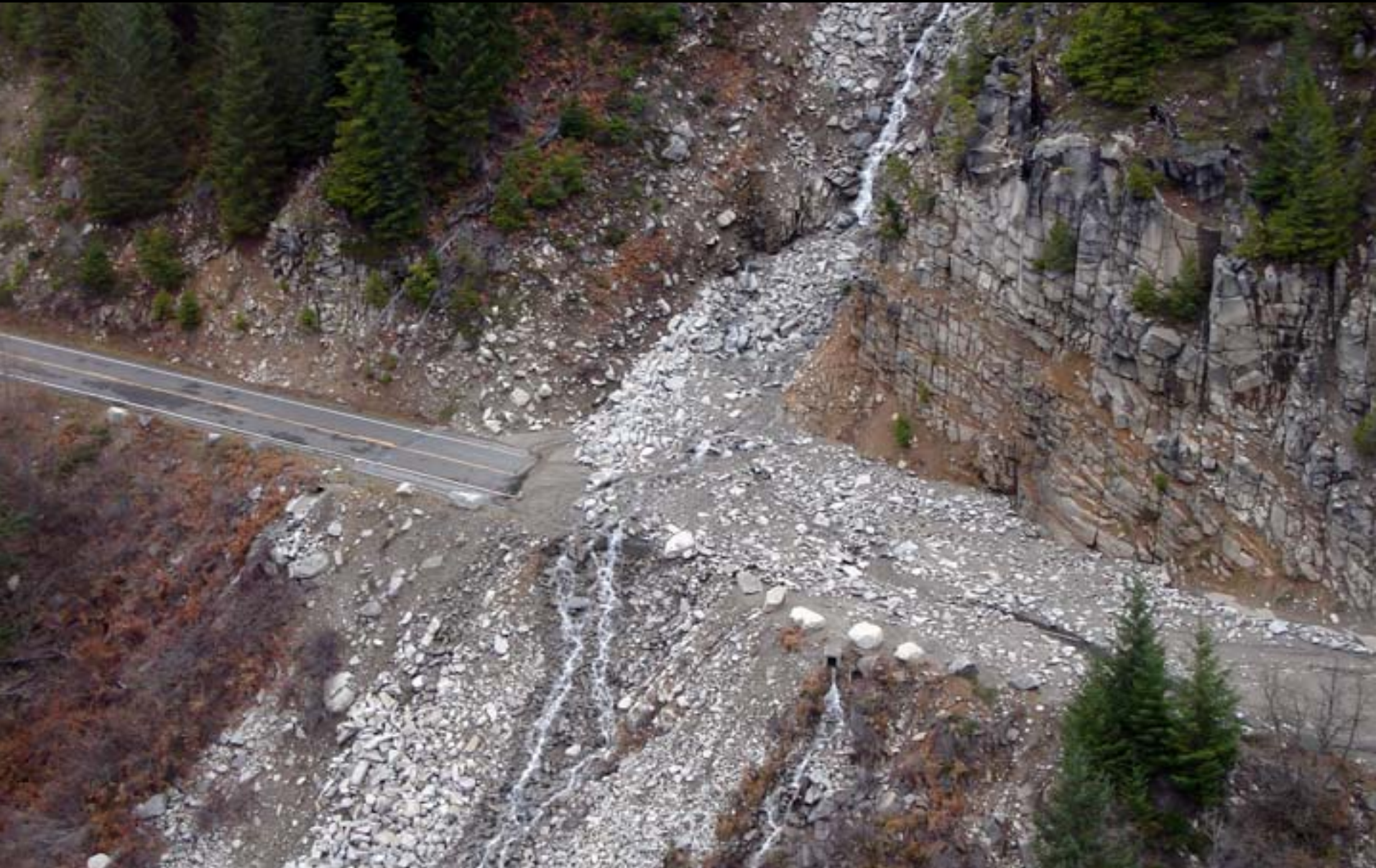
Landslide below Stevens Ridge in Stevens Canyon
