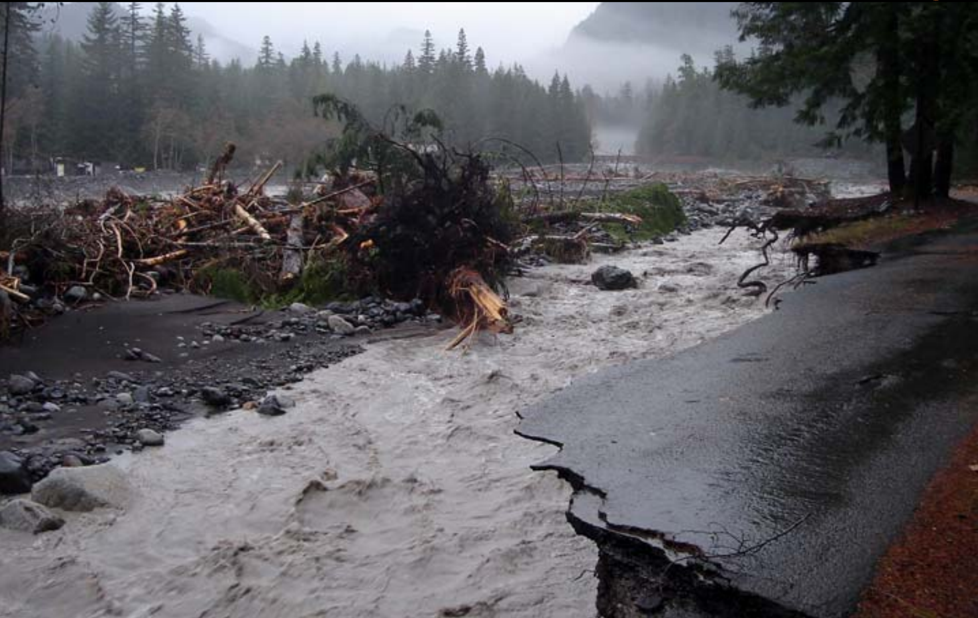
Washout in front of the Community Building at Longmire
