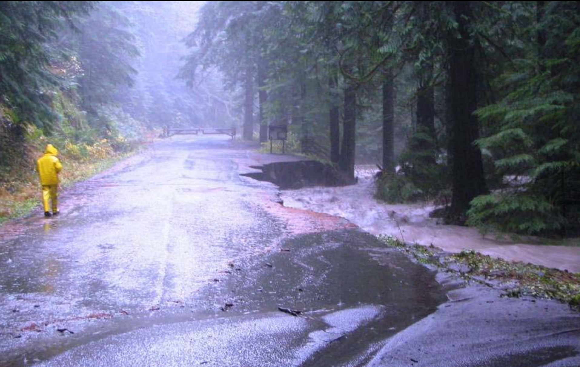
Washout at the beginning of the Westside Road
