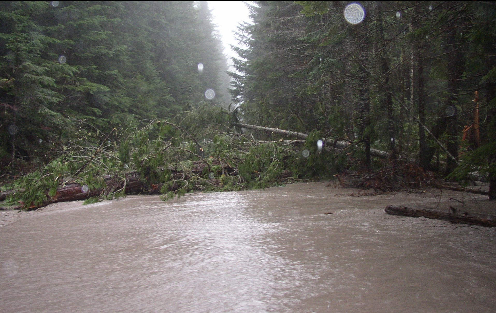
Flooding and fallen trees on Highway 410 near the park entrance
