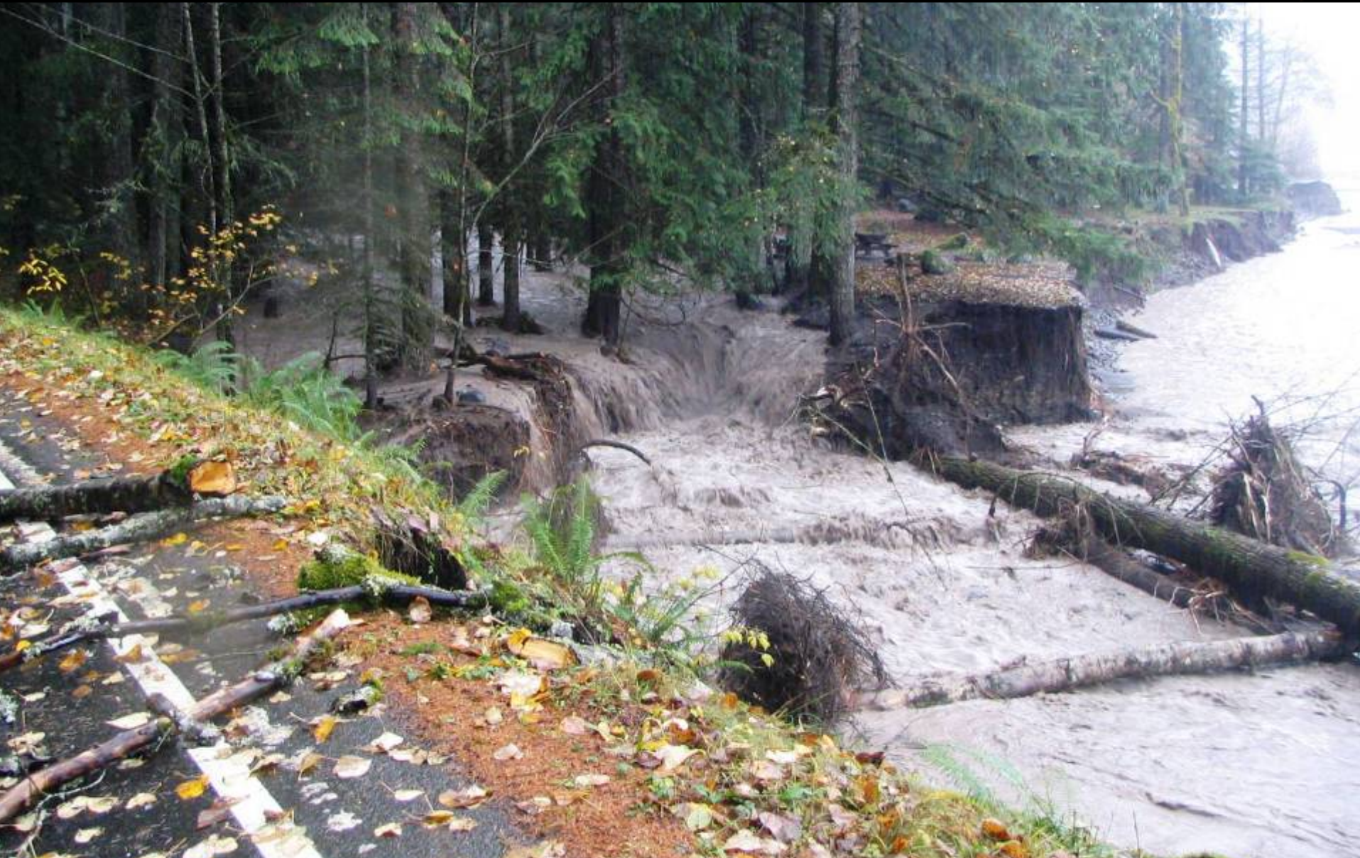
Water flowing through the remains of the Sunshine Point Campground
