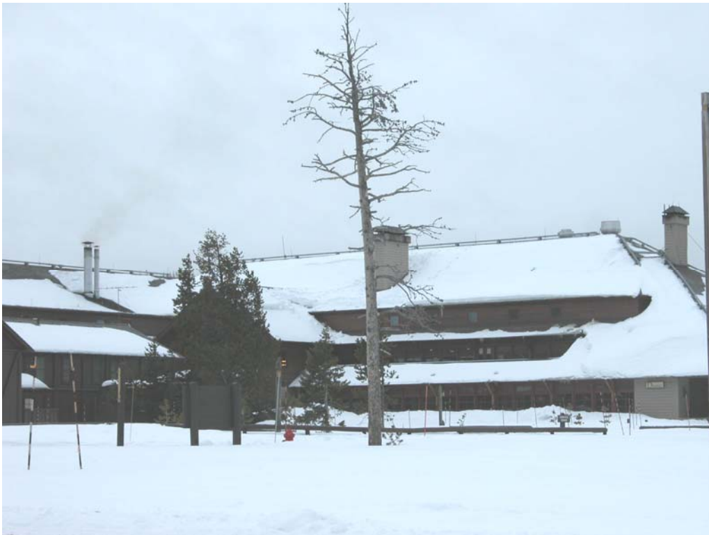
View of Snow Lodge to the south of the monitoring shelter. Smoke can be seen raising from the boiler room. The two large stacks are from the gas-fueled public area fireplaces which do not produce visible plumes. During the evening, smoke can be seen coming from the kitchen vents that are on the far side of the roof, right side.
