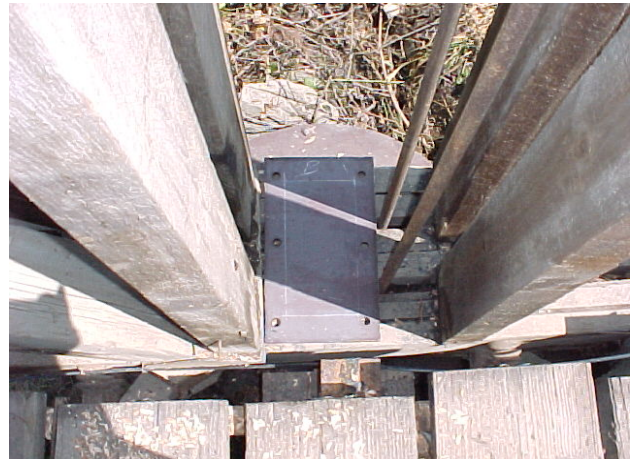
Figures 23 & 24 Setting the foot plate for the steel.
