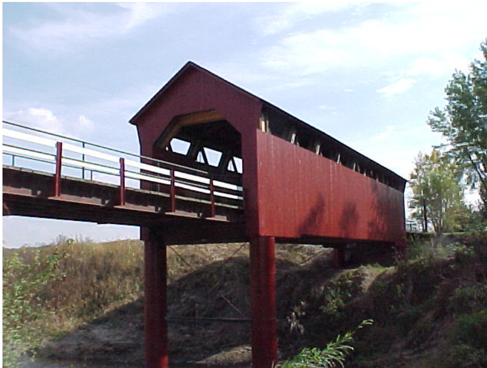
Figure 20 Hammond Bridge, rehabilitation finished, looking southeast.
