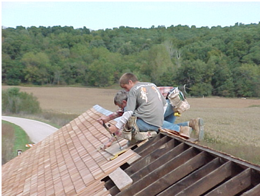
Figure 40 Re-roofing with cedar shingles.
