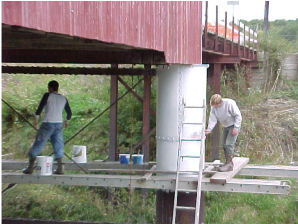
Figure 33 Priming a caisson/cylinder pier.
