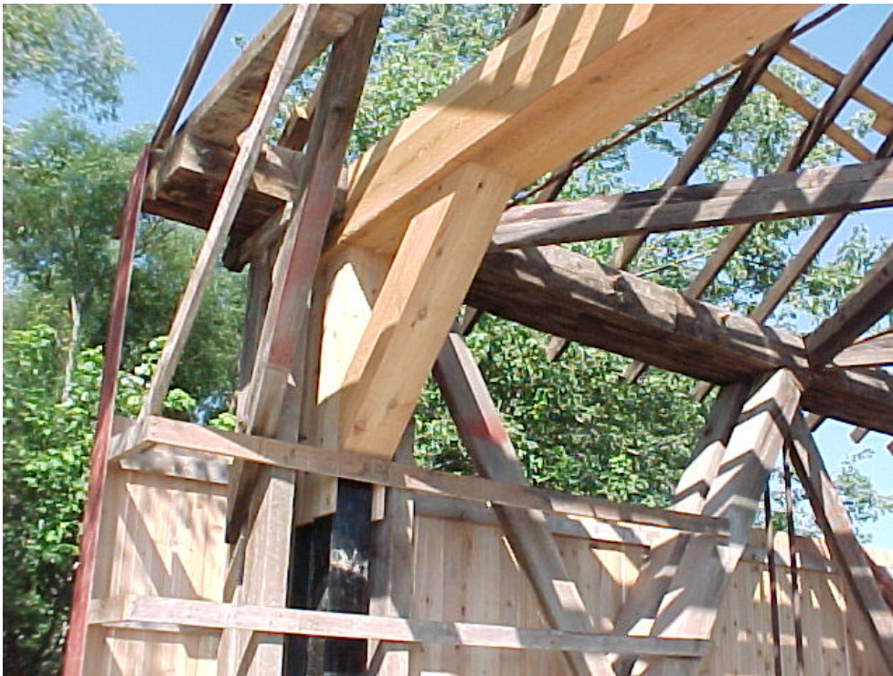
Figure 28 Cedar lumber hides the steel.
