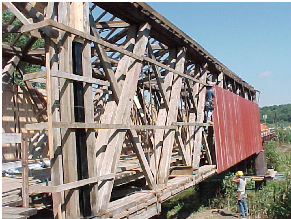
Figure 38 Replacing the siding.
