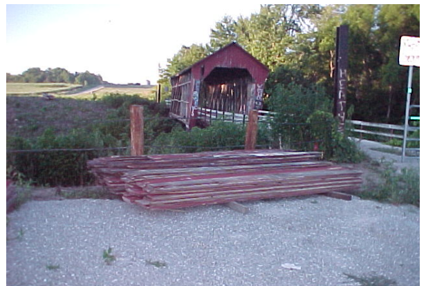
Figures 35 & 36 Removing and storing siding.
