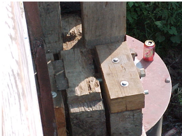
Figures 30 & 31 Floor beam and pier trouble spots.
