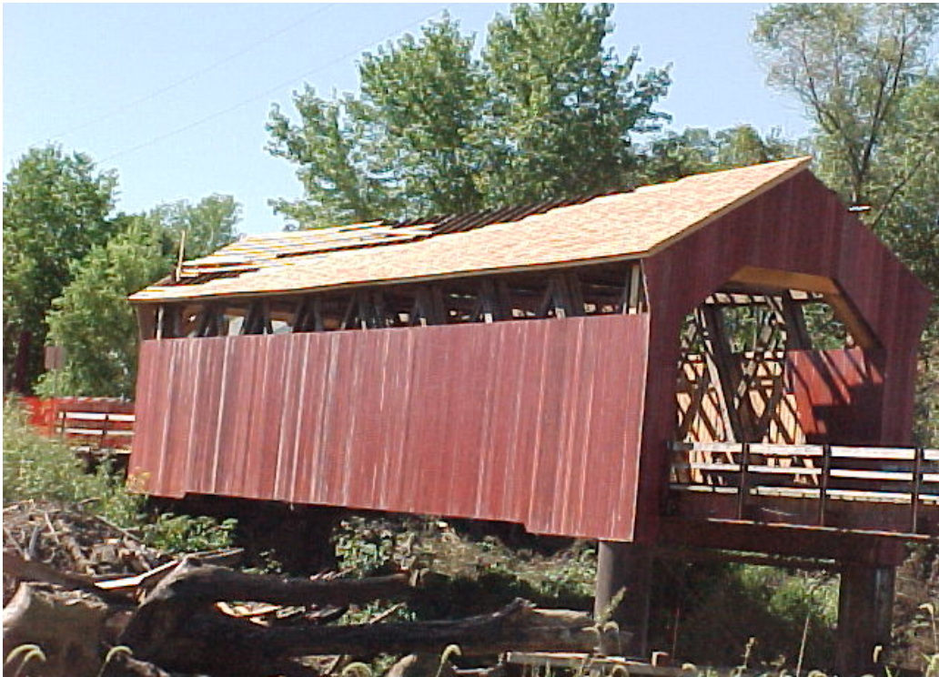
Figure 39 The roofing in process.
