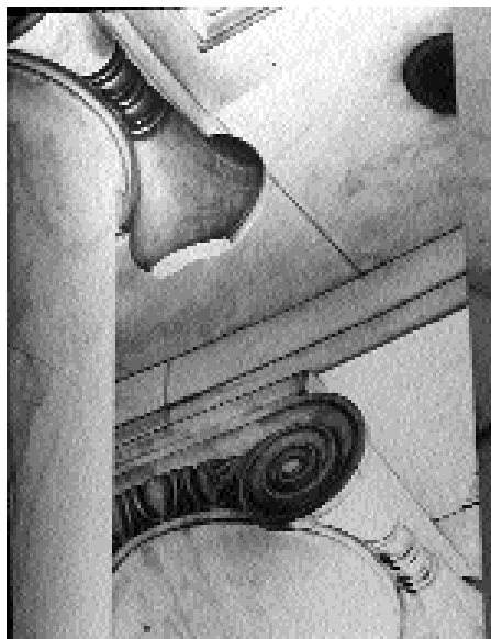
View of a broken volute on an interior column at the Jefferson Memorial, c. 1962.
