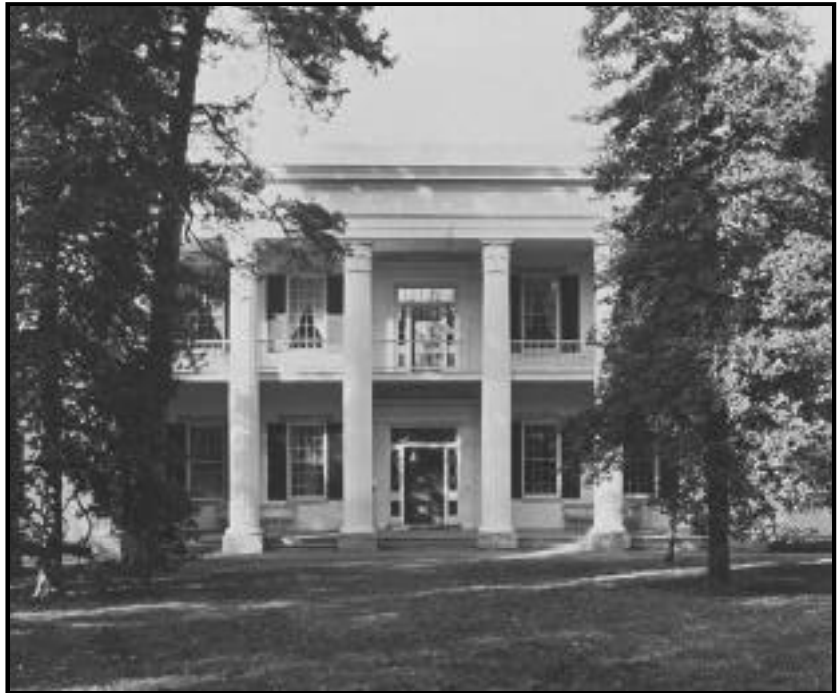
Prior to the April 1998 tornado, The Hermitage mansion was framed by an 1838 carriage drive lined with mature Eastern Red Cedars. Photo courtesy The Hermitage.
